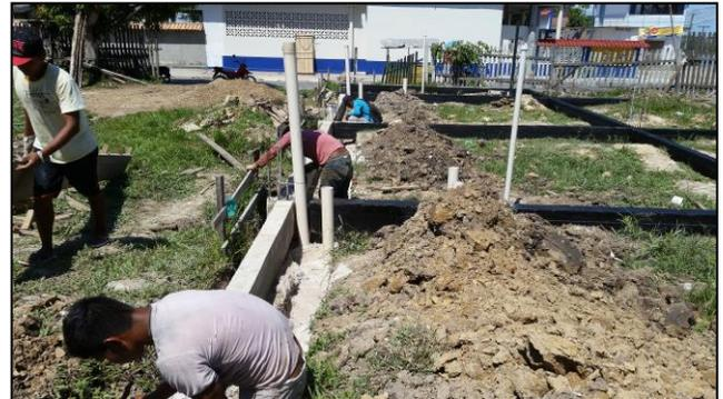
Church storefront construction project--foundation and plumbing in place before pouring the floor.
