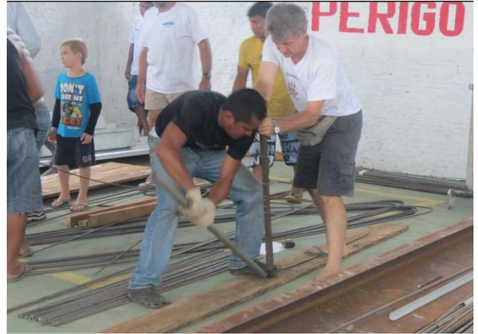
**Bending rebar to go into concrete forms.**
