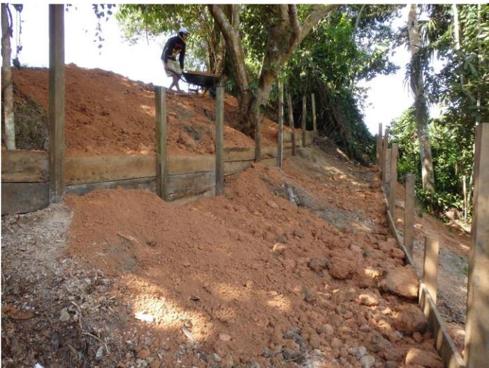
**Mudslide in the back yard being fixed by creating a terrace.**
