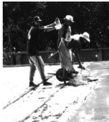
This construction crew finished the concrete pillars and laid the concrete roofing. Their workdays started at dawn when the temperature was cooler.
