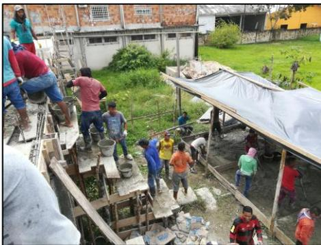
These photos show the preparation of the second floor and the concrete being poured bucket by bucket, a task that took 16 hours. We will be delighted when the project is finished.
